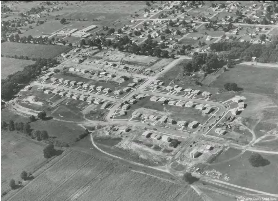
Figure 18. A c.1950 aerial photograph of the Southland Village residential subdivision under construction. 23
