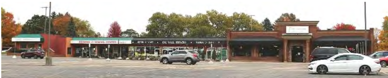
Figure 10. Several Bloomfield Shopping Center buildings located on Portage Street on the block between Dorchester Avenue and Bloomfield Avenue, view east from sidewalk along Portage Street. The address range for these buildings is 4203-5217 Portage Street.
