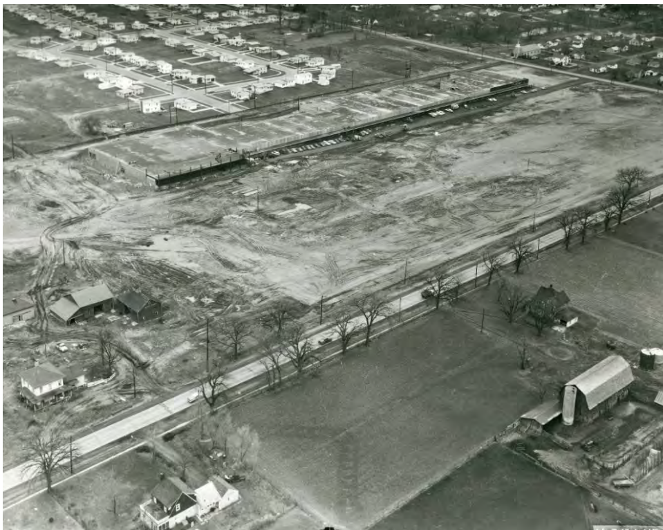
Figure 19. A c.1958 aerial photograph of the Southland Shopping Center under construction at S. Westnedge Avenue and W. Milham Avenue. Note the recently constructed Southland Village subdivision in the background. 24
