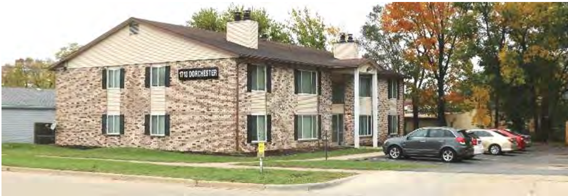
Figure 15. Multi-family residential building at 1713 Dorchester Avenue, constructed c.1970, view northwest from Dorchester Avenue between Portage Street and Moreland Street.
