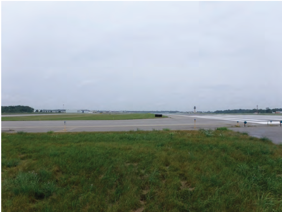
Photo 10. Existing runway and taxiway, southern end of APE, facing northwest
