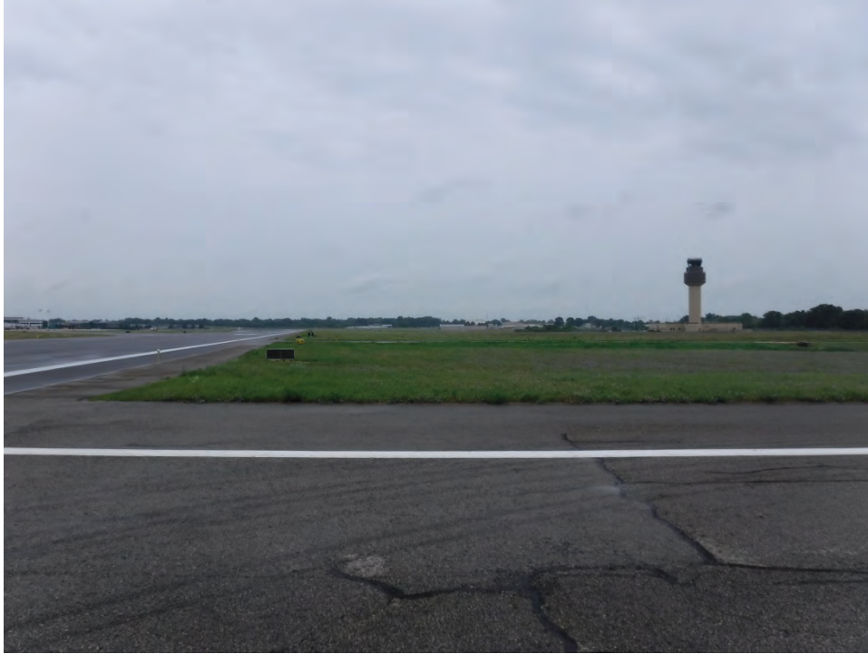
Photo 11. Conditions within central APE along existing runway, facing northwest
