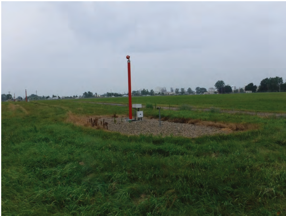
Photo 6. Existing approach light in southern end of APE, facing southwest
