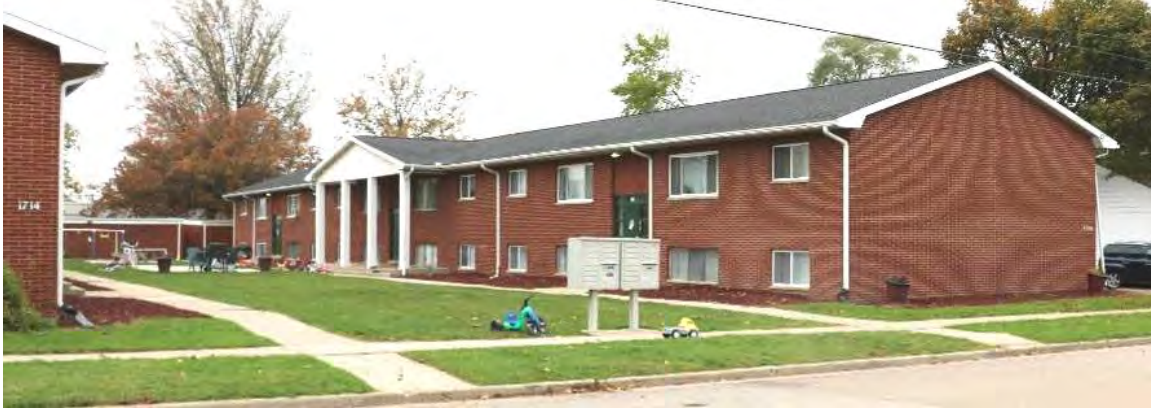
Figure 14. Bloomfield Apartments at 1706-1714 Bloomfield Avenue, constructed in 1964, view southwest from Bloomfield Avenue between Portage Street and Moreland Street.
