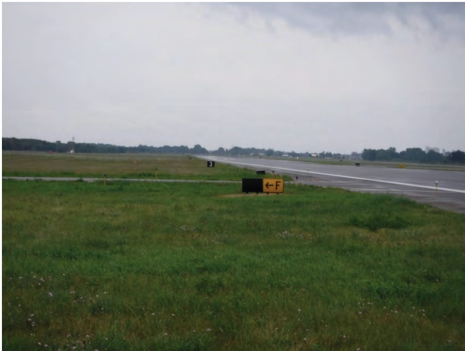
Photo 12. Conditions within central APE along existing runway, facing southeast
