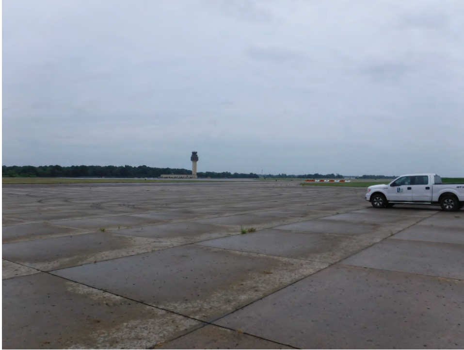
Photo 17. Northern portion of APE within existing infrastructure, facing southeast
