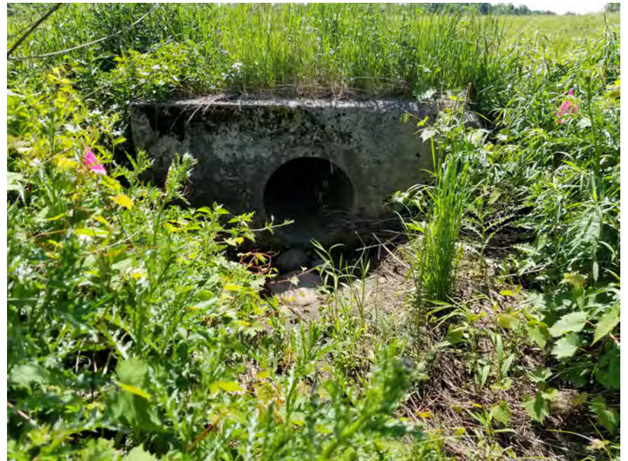
Photo 16. Wetland 2, Culvert headwall.. View to the east. (June 07, 2019).
