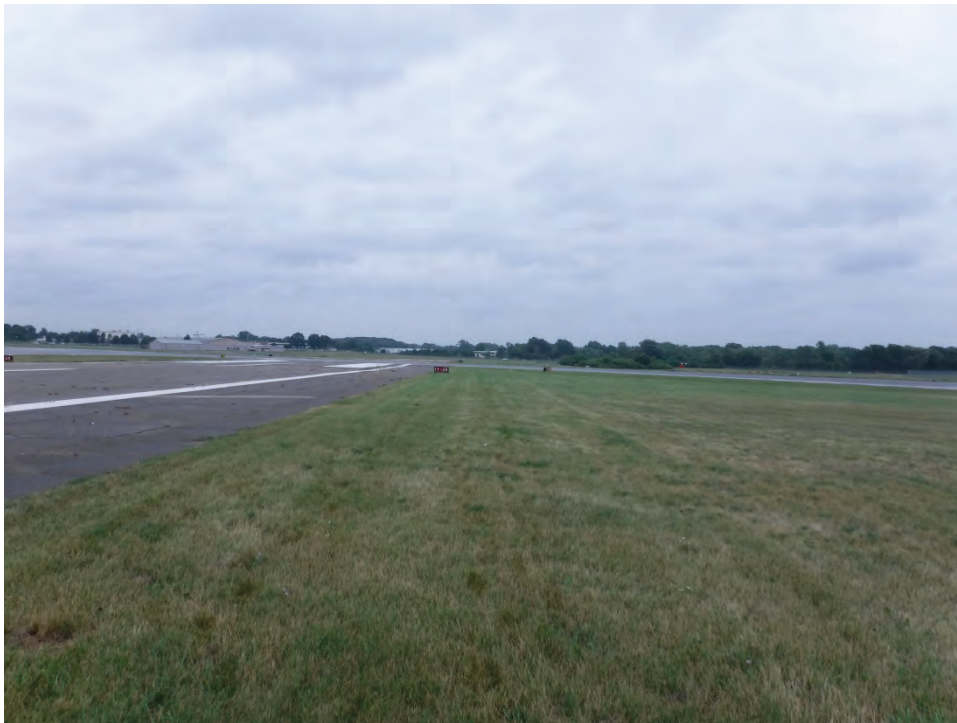
Photo 14. Conditions along existing runway in northern APE, facing northeast
