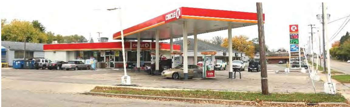
Figure 11. Contemporary infill development at 4117 Portage Street, view southeast from the intersection of Portage Street and Golfview Avenue.
