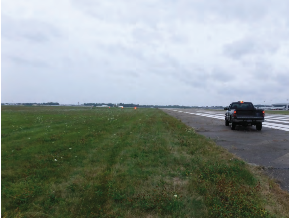
Photo 13. Conditions along existing runway in northern APE, facing southwest
