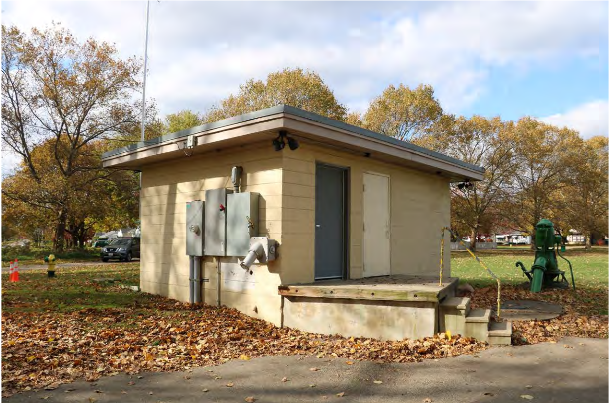
Figure 5: The east and south elevations of the c.1970 utility building located at the southwest corner of Emerald Drive Park.
