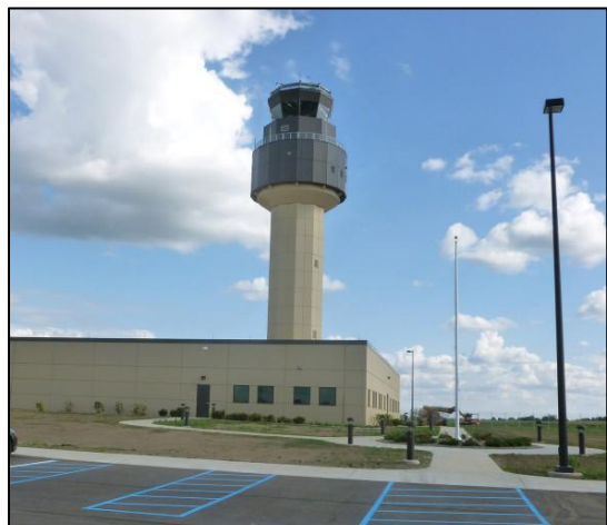
AZO Airport Traffic Control Tower
